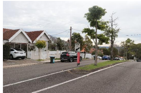
Figure 83: Divided road at north end of Lang Street.
