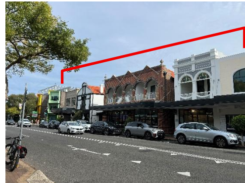
Figure 118: View of central portion of Military Road, from left to right – 743, 741, 739, 737 Military Road.
