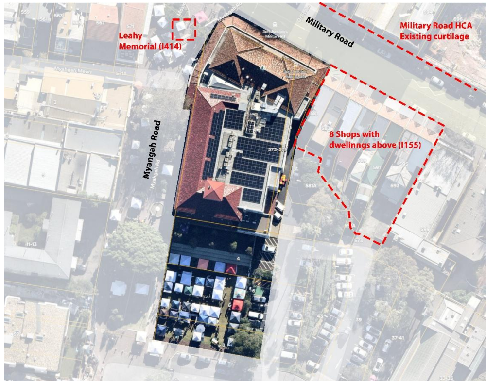
Figure 127: Aerial photograph of the Mosman Civic Centre. (Source: Nearmap with NBRS edits)
