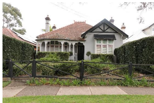
Figure 94: Contributory-1 place, 3 Lang Street.
