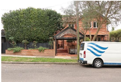
Figure 91: Neutral-4 place, 17 Lang Street.
