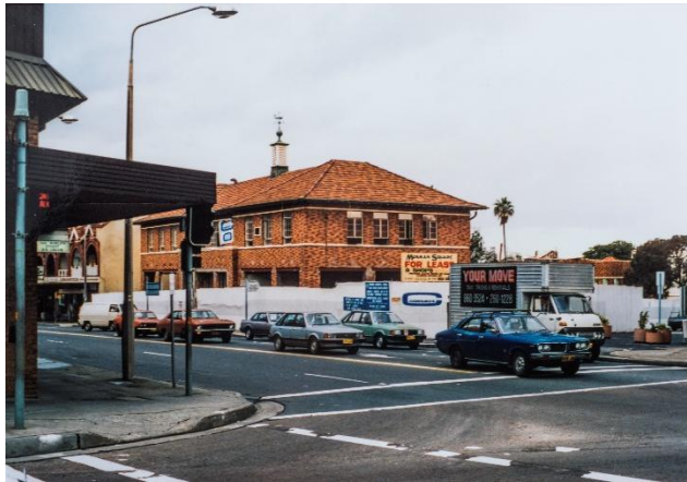
Figure 18: Mosman Council Chambers under construction, with the retained interwar portion of the building shown, taken in 1987. (Source: race Mosman Digital Archive)
