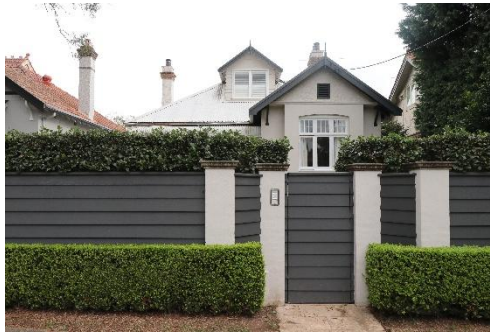
Figure 95: Contributory-2 place, 5 Lang Street.
