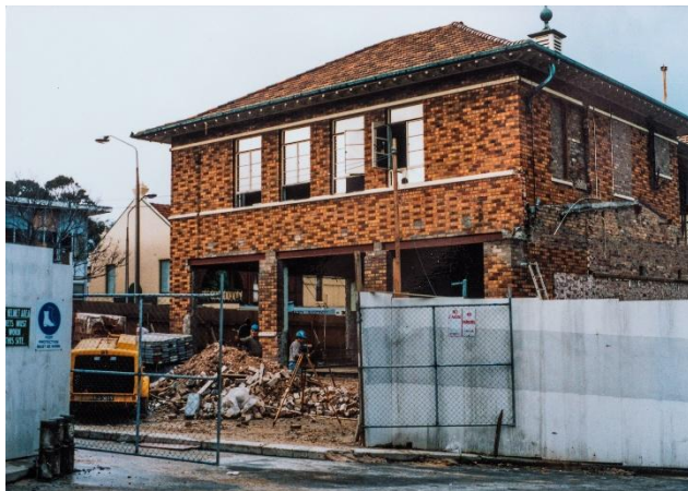
Figure 19: Mosman Council Chambers under construction, with the retained interwar portion of the building shown, taken in 1987. (Source: race Mosman Digital Archive)
