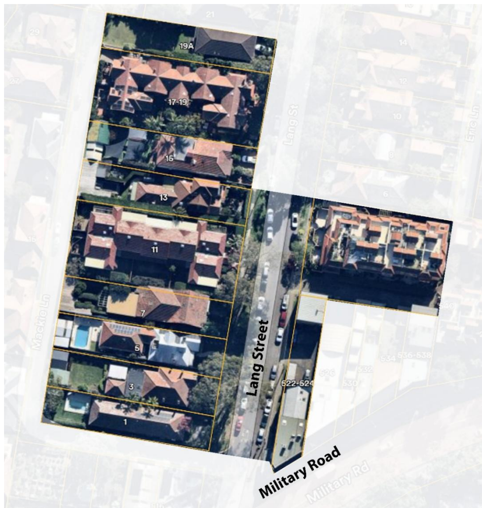
Figure 84: Aerial view showing the southern portion of the Lang Street HCA. (Nearmap with NBRS edits)
