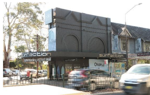
Figure 86: Shop fronts to 522-524 Military Road.
