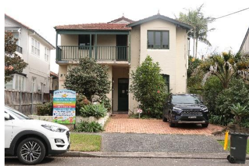
Figure 90: Neutral-4 place, 15 Lang Street.
