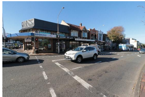
Figure 100: Row of shopfronts at the Military Road intersection, included in the Military Road HCA.
