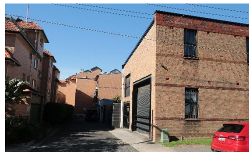
Figure 88: Warehouse at rear of 522-524 Military Road, fronting Lang Street, Mosman.
