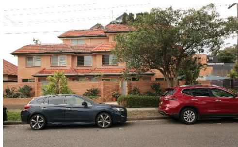
Figure 87: Detracting development at 2 Lang Street, Mosman.
